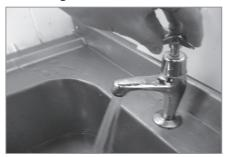
Fill sinks with clean water and empty to flush through unit. This keeps freshwater in tank. Always ensure water level is reaching wheels/drum.
